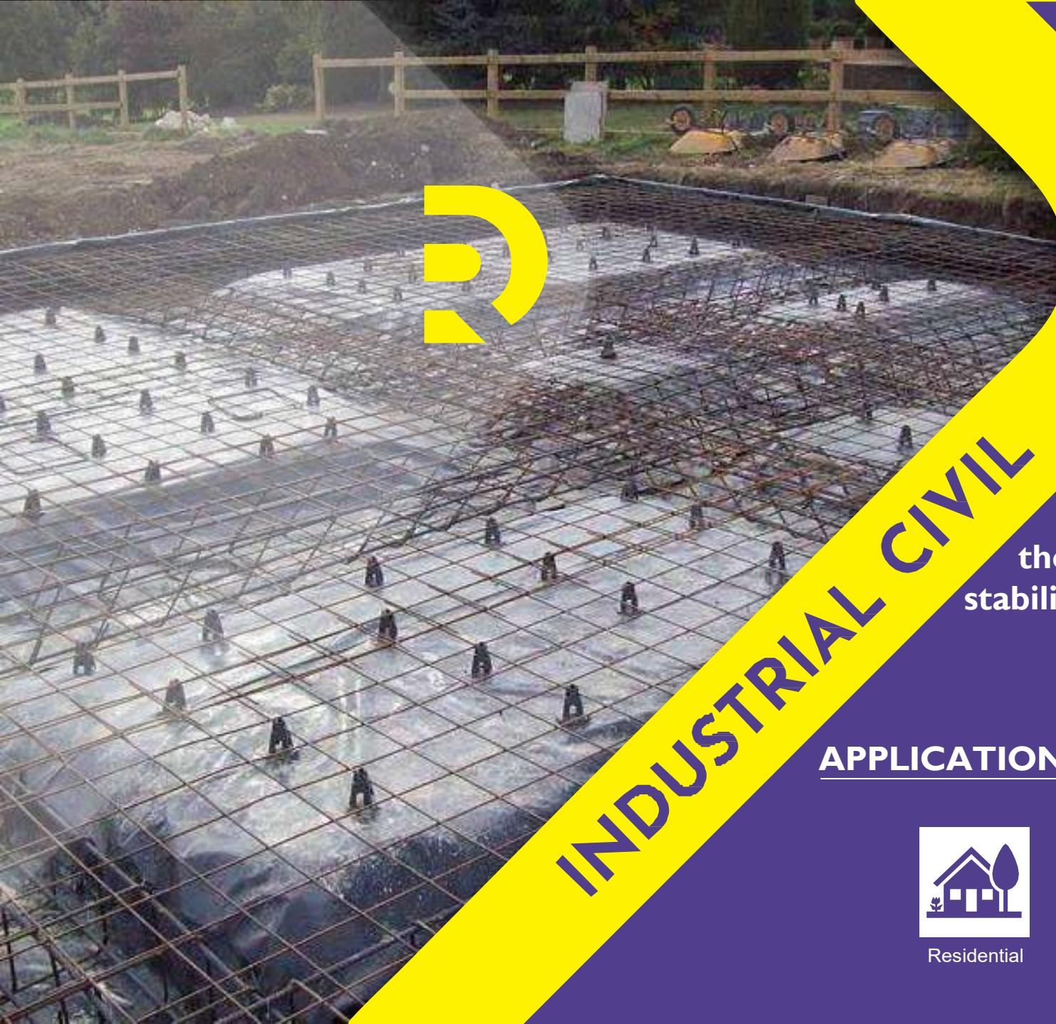
A **raft foundation**, also known as a **mat foundation**, is a type of foundation used to distribute the load of a structure over a large area of soil.
